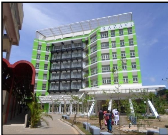
Rasavi Building- National Cancer Institute - Maharagama
