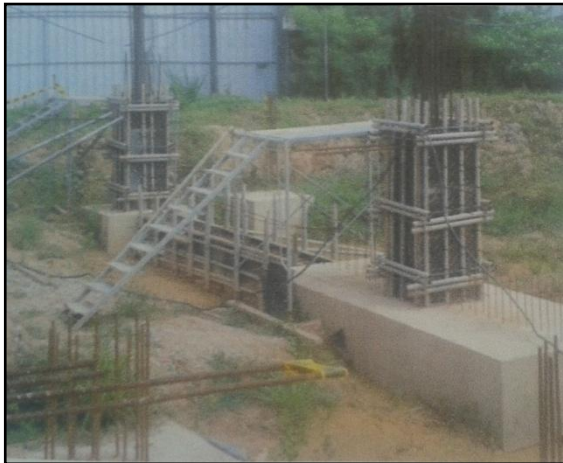
Construction Works at National System Control Modernization Centre - Sri Jayawardhanapura
