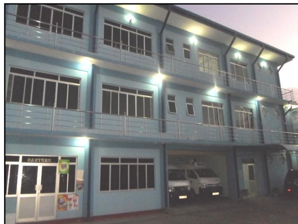
Kaluwanchikudy Hospital - Batticaloa
