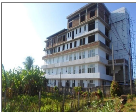
Building Complex for Professorial Unit at Eastern University - Batticaloa
