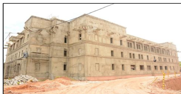
Communication Building and Signal Tower
