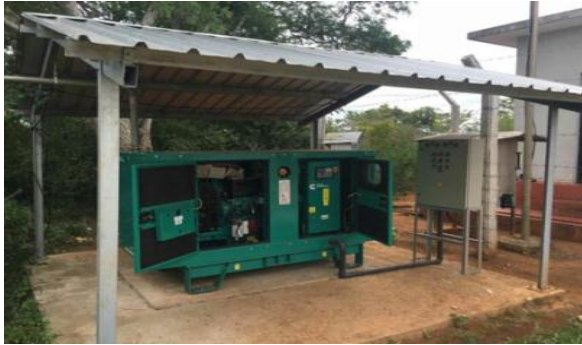
Generator installation at Thanthirimale
