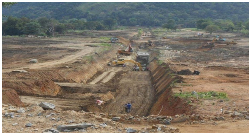
Kuda Oya Reservoir Dam – Core Trench filling
