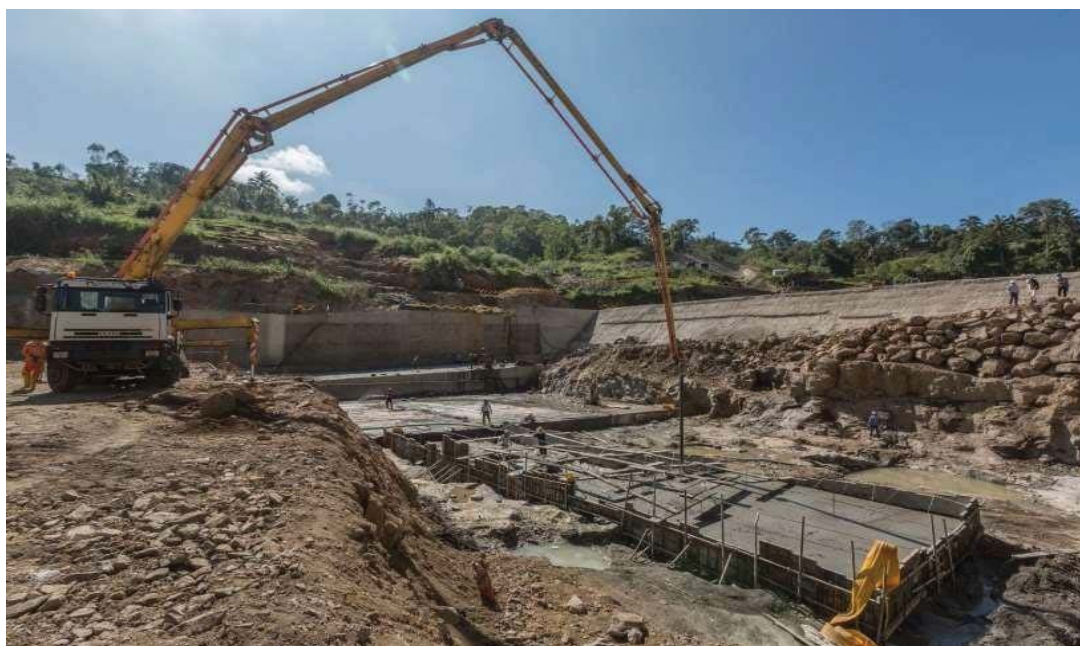
Puhulpola Dam Foundation Excavation on going
