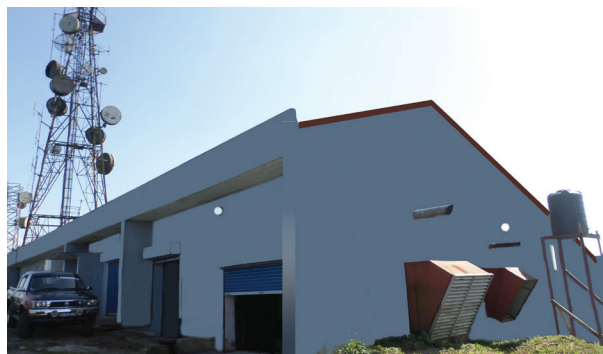
Renovated Karagathenna Transmission Station
