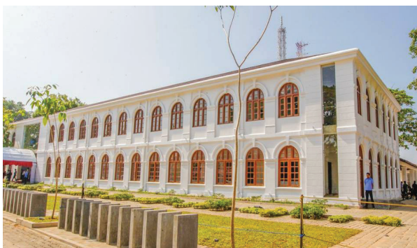
New Administration Building
